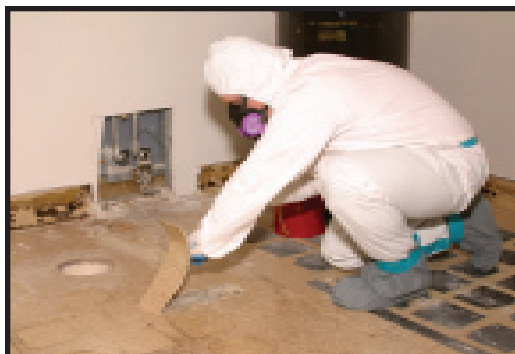
Prying up a section of flooring
